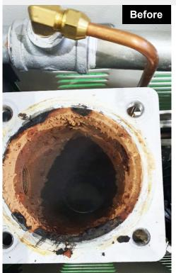
Scale was not removed before Vulcan S10 was installed.
